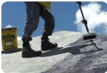
YouTube Palco Waterproofing Bituminous primer on concrete
